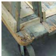
Wood—splinters and rots
